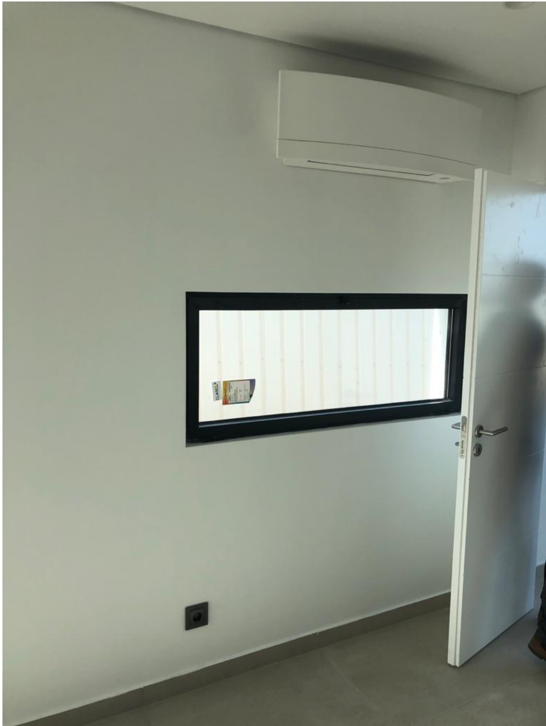
Picture 6 – Office area
